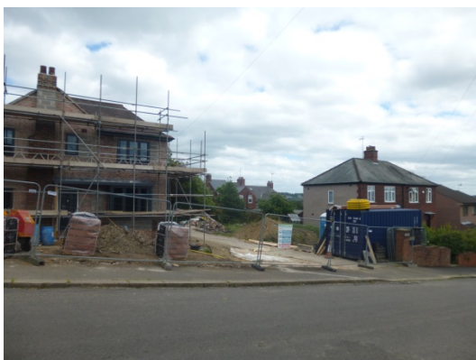
Photo taken from Cavendish Street North highway facing south east towards site
