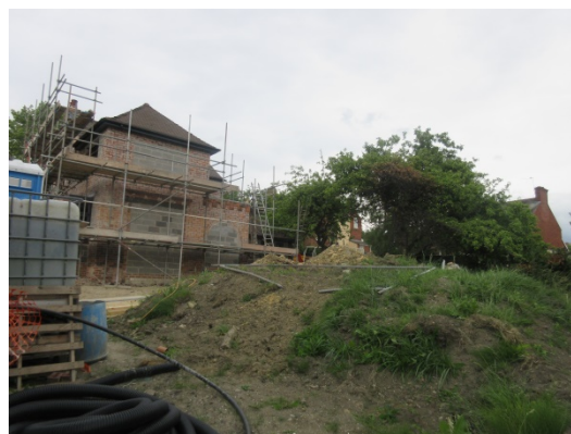
Photo taken facing north east towards the side elevation of No 12 Cavendish Street North
